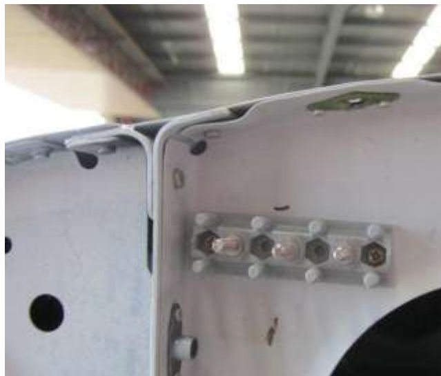
Figure 5 - Terminal Strip installed (item 2).
